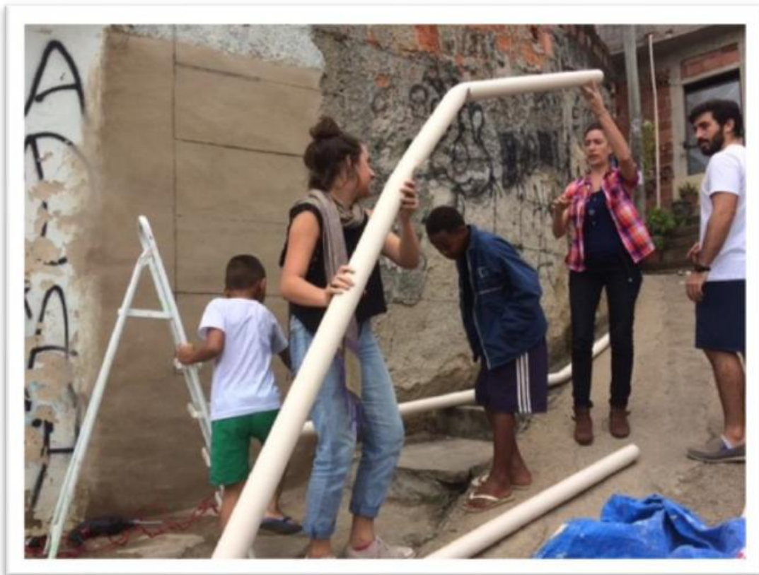
Figure 4: Attaching the tubes at the wall/Morro do Palácio, 2017
